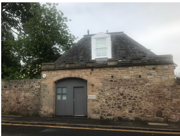
Figure 3: The Pump House on Blackford Avenue, 2021.
