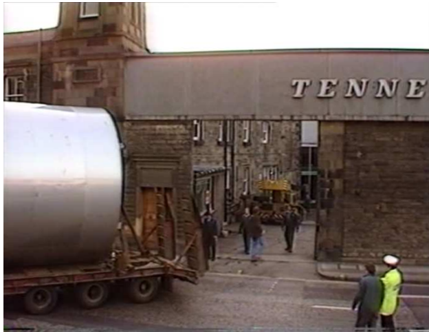
Figure 4: Roseburn Terrace gate open for delivery of a new vessel.
