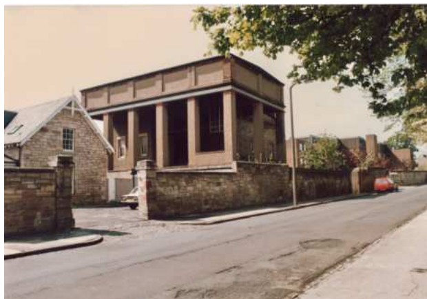
Figure 1: Water tank and well situated on Grange Loan, 1986.
