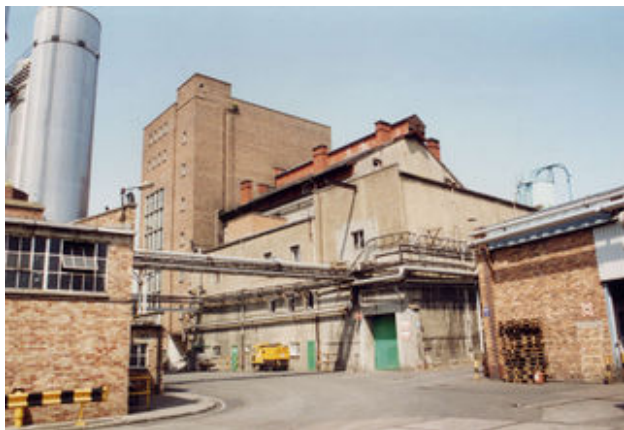
Figure 5: View of the Lager Building from Russell Road gatehouse. The boiler house is on the left and keging hall on the right.
