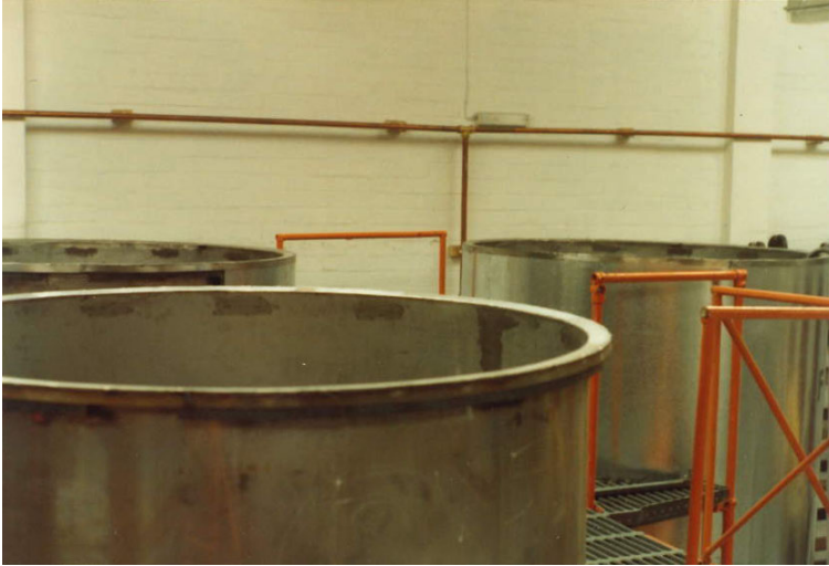
Figure 5: There were five 15-barrel open fermentation vessels. These were cleaned by hand by getting inside with a bucket of caustic, rubber gloves and safety glasses! There were actually six of these vessels, however one was used as the hot liquor tank and whirlpool.
