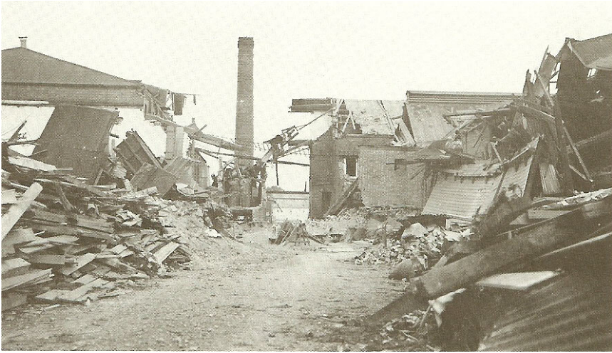
Figure 4: Bomb damage after the 1942 raid.
