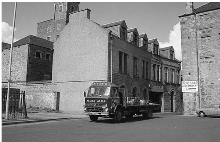
Figure 10: The old dray loading arrangements were made from in front of the office block
