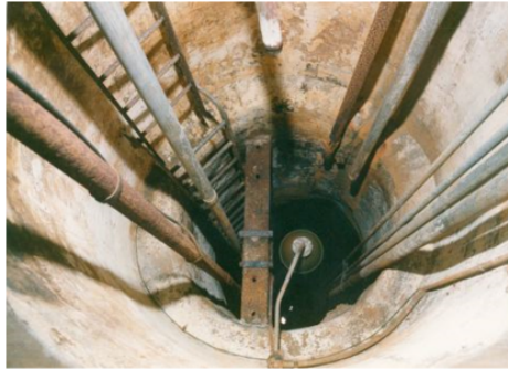
Figure 5: The interior of the brewery water storage well. This was not one of the two productive wells.
